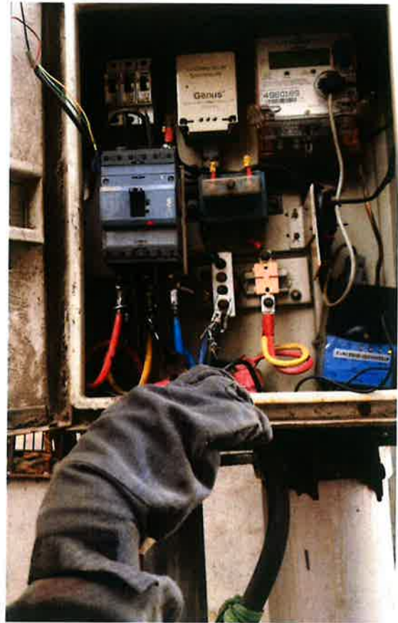
Hooking removal from Meter Pillar Box
